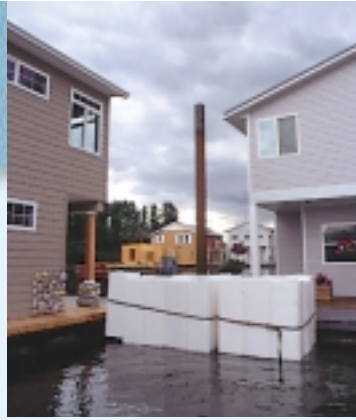
White bead foam encapsulated with 7 mil plastic sheeting is available from many marine retailers.
